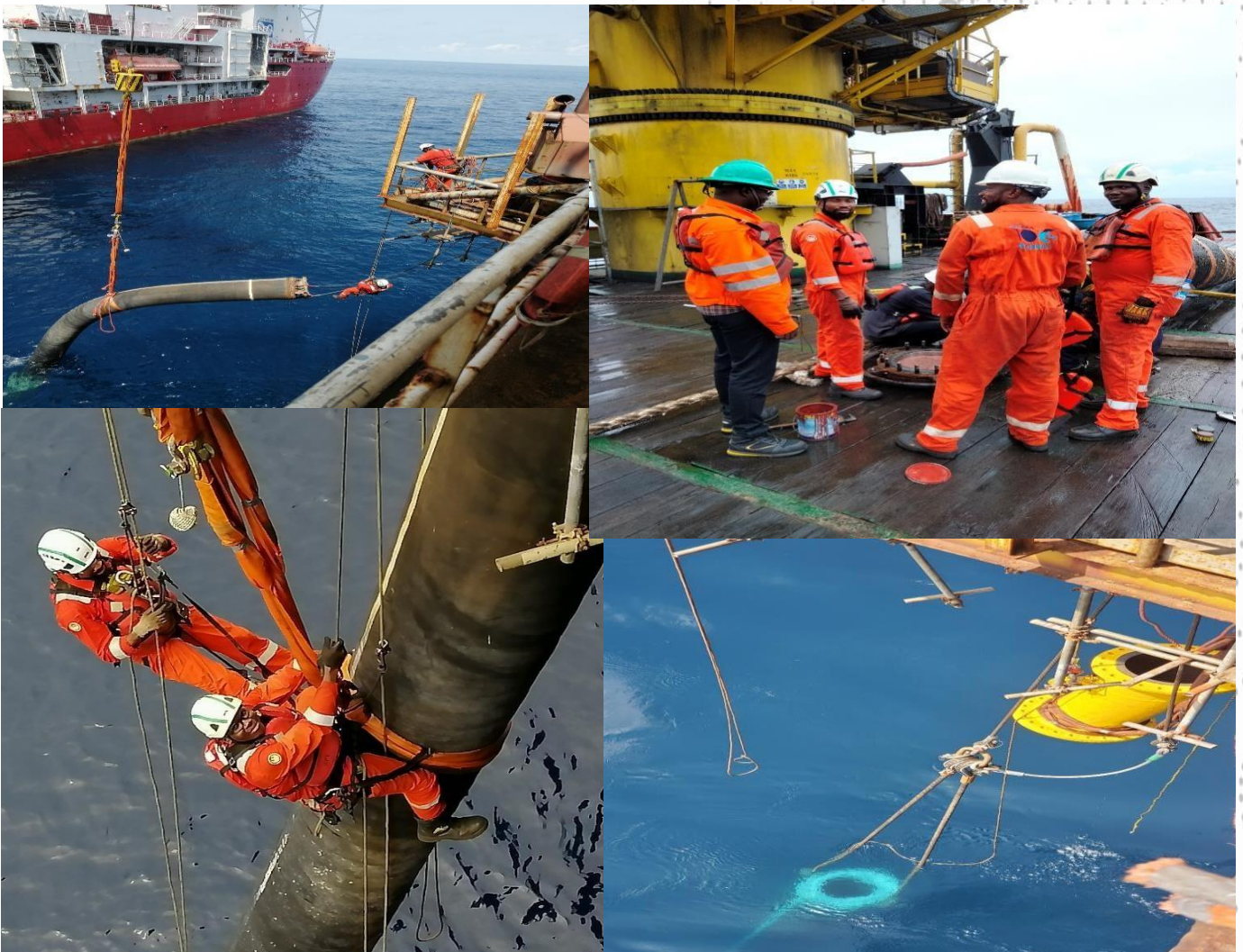
The team installing a 24 inch export hose at OML 119
